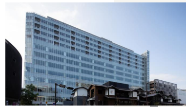
Minaka Odawara Building
